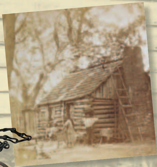
Cabins were usually made of small logs, about 10 to 20 feet square. Often, two or three families shared a cabin.
