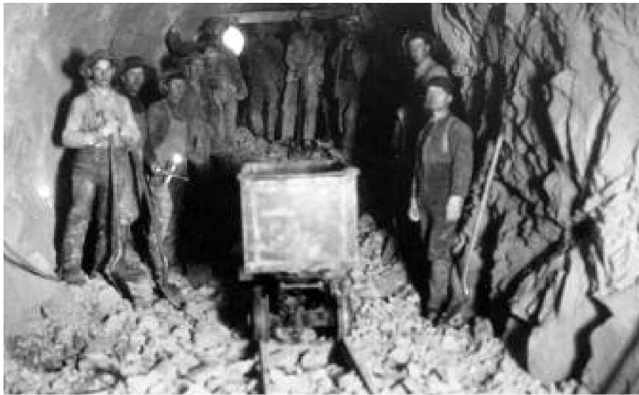
Men dug out a tunnel under the mountains to divert water from the Strawberry River while the dam was being built.
