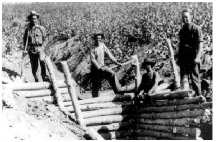
CCC workers in Hobbie Creek Canyon east of Springville worked to build a log dam for soil conservation.
