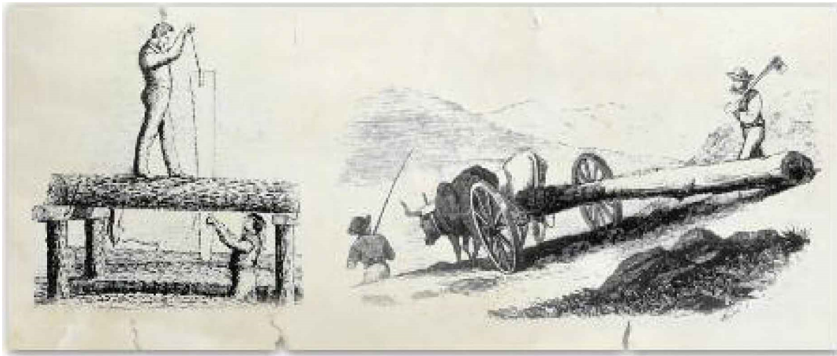
Pit saws were used to saw logs into boards. One person stood down in a pit and helped move the saw up and down.
