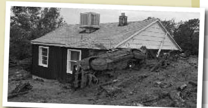
In Farmington, a car lies sideways in a wall of mud that caused major damage to 30 homes in 1983. About 2,000 people were moved to safer ground.
