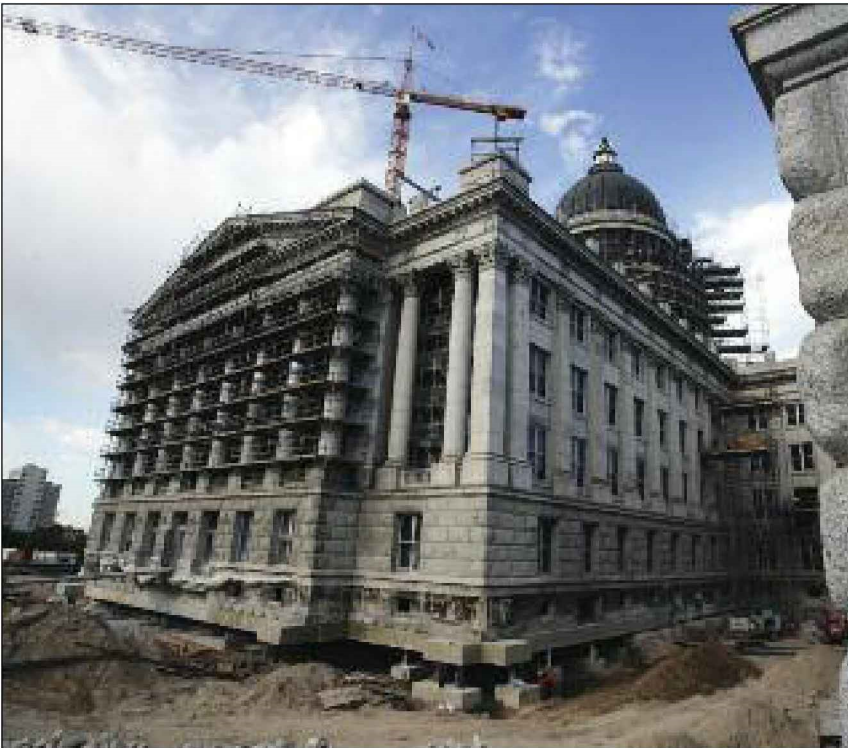
In 2004 the Utah State Capitol building was closed for renovation. Large shock absorbers were placed under the building to make it more stable in case of an earthquake. Construction was completed in 2008.
